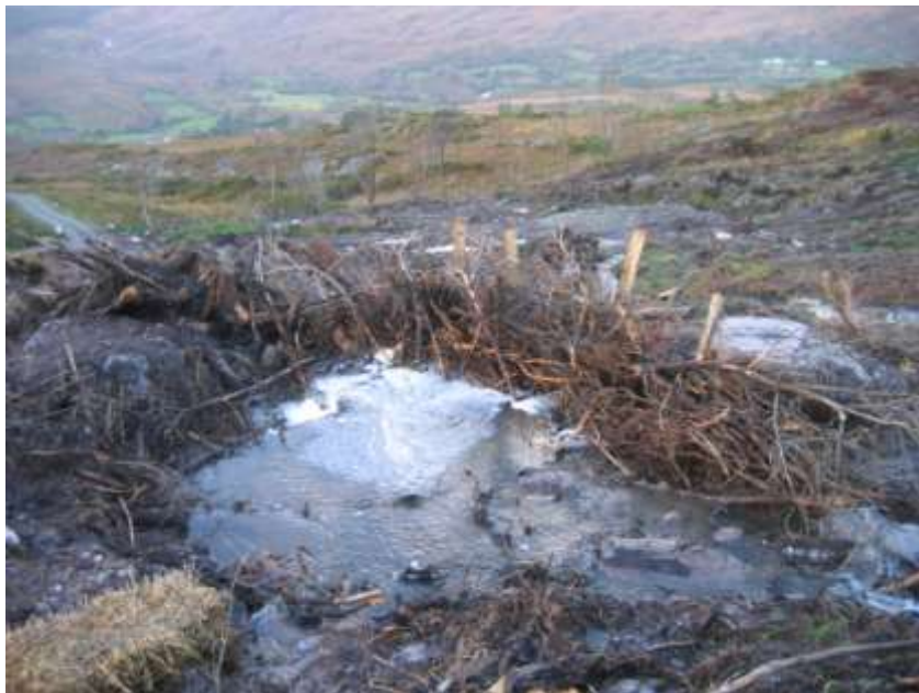
Silt trap constructed by contractors is commendable, but will require maintenance.
